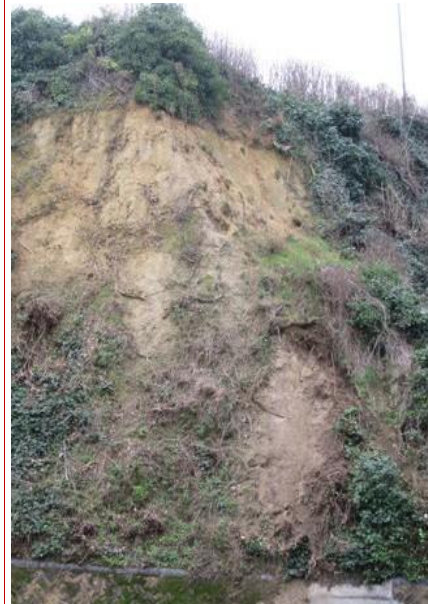
Area B south side of Fraser Road
