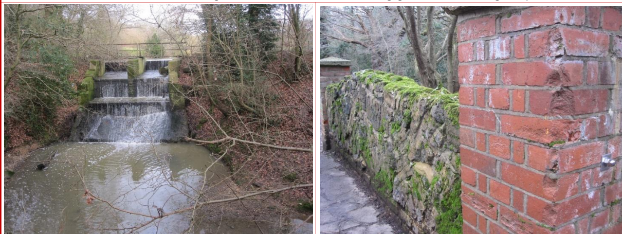
East end: London Clay beneath the weir from Jack's Lake; over-burnt bricks on the bridge over Pymms Brook coming from Jack's Lake – an indication of local brickmaking probably from the silty Claygate Member.
