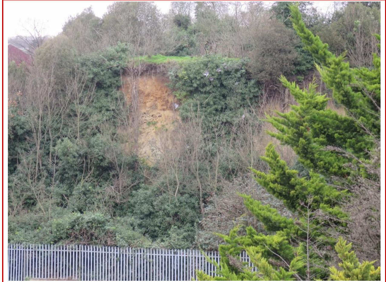
Area A from Erith railway station, February 2016. Photo: Laurie Baker
