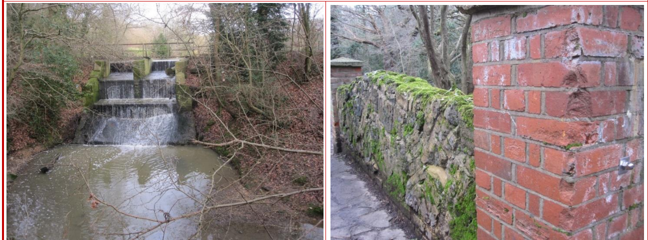
East end: London Clay beneath the weir from Jack's Lake; over-burnt bricks on the bridge over Pymms Brook coming from Jack's Lake – an indication of local brickmaking probably from the silty Claygate Member.
