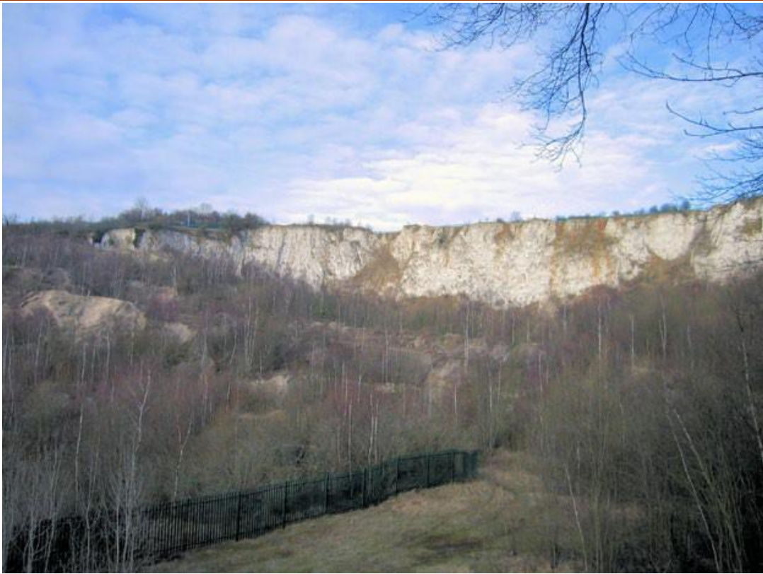
View of north east quarry face
